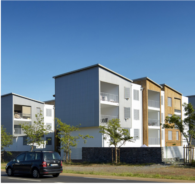
© Co-Architectes, Les Mahots
