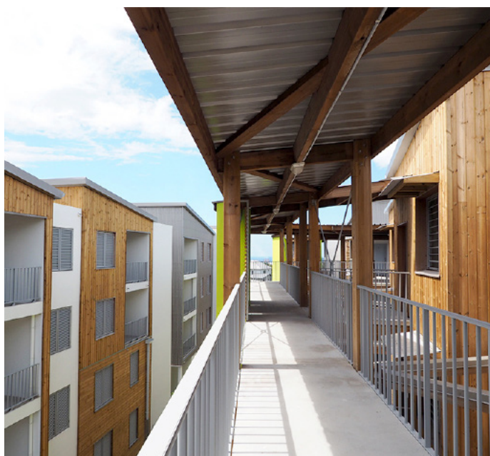
© Co-Architectes, Les Mahots
