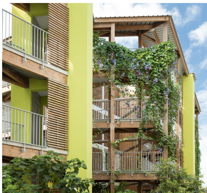
© Co-Architectes, Les Mahots
