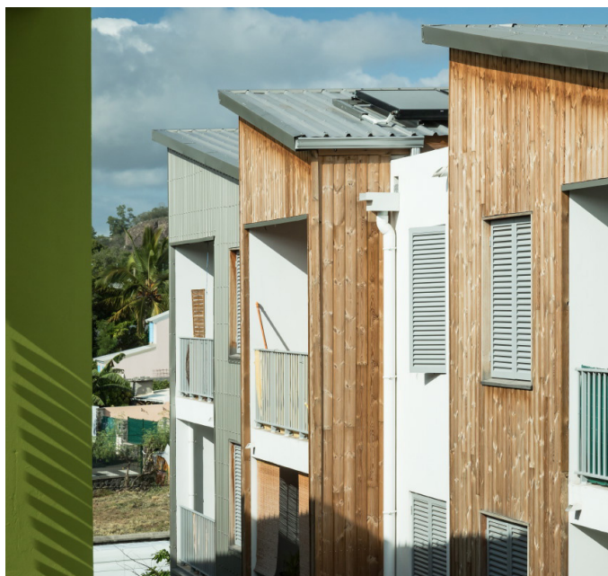
© Co-Architectes, Les Mahots
