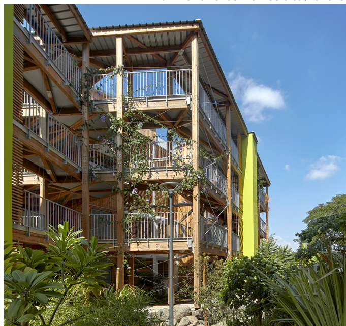
© Co-Architectes, Les Mahots
